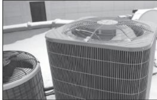
Air conditioning systems
