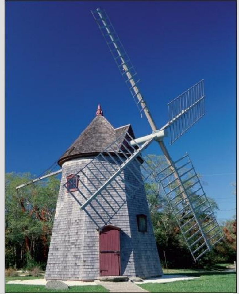
A restored windmill in Brewster, MA, that was used in the 1800s to grind grain. (Note that the blades must be covered to function.) Modern “windmills” that generate electricity are more properly called wind turbines .
