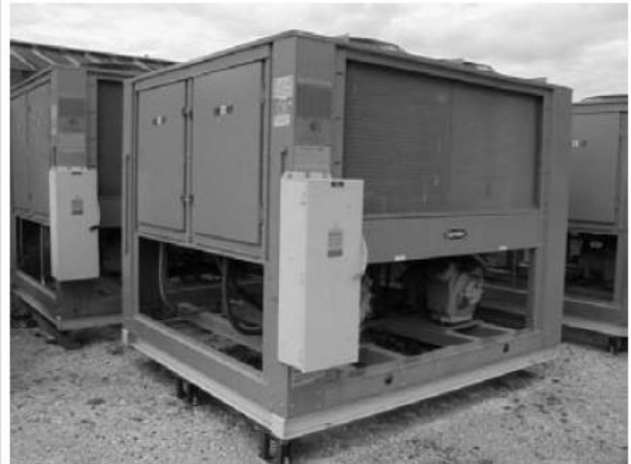
Figure 3.18 A typical air-cooled condenser
